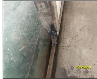
Photo of the inside of the main production hall Sliding door was melted with door frame before audit.JPG
